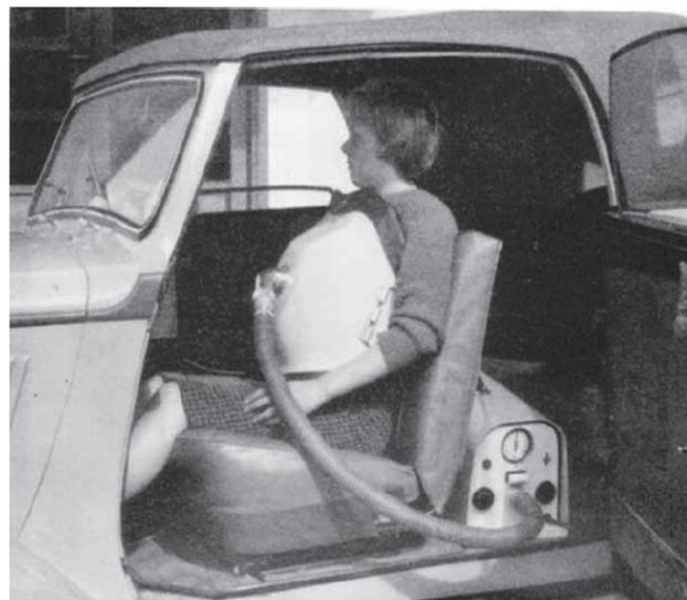
Fig 2. Cuirass shell ventilator.
